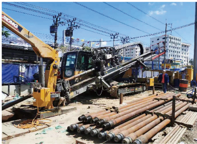
XZ1350 working for gas pipeline construction in Thailand
