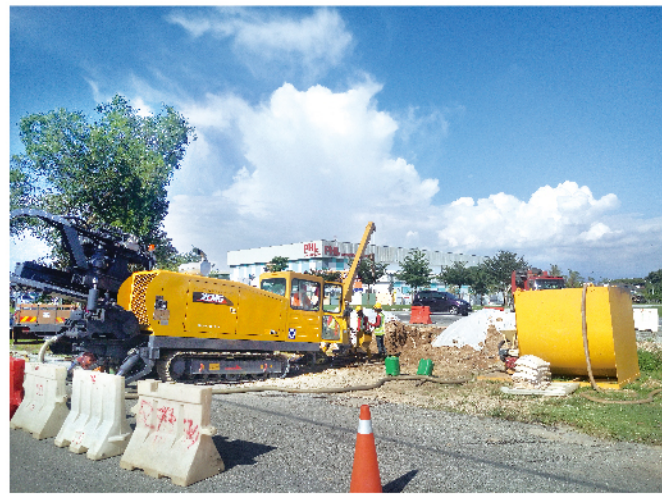
XZ450 working for the construction of natural gas pipeline in Malaysia
