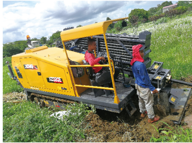
XZ320E working for the communication pipeline construction in Philippines
